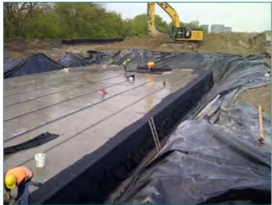
Underground Stormwater Management Chamber
