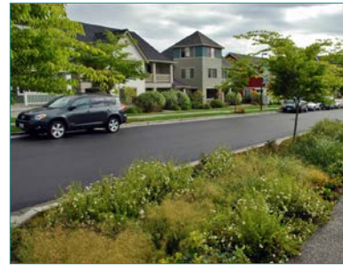
Swale in Boulevard (LIDs)
