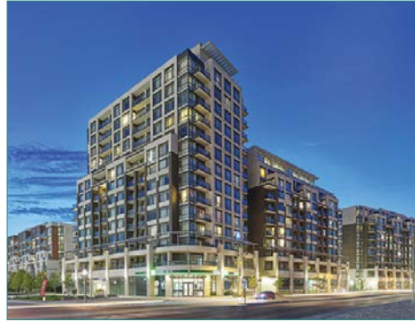
High-rise Apartments (12 + Storeys)
